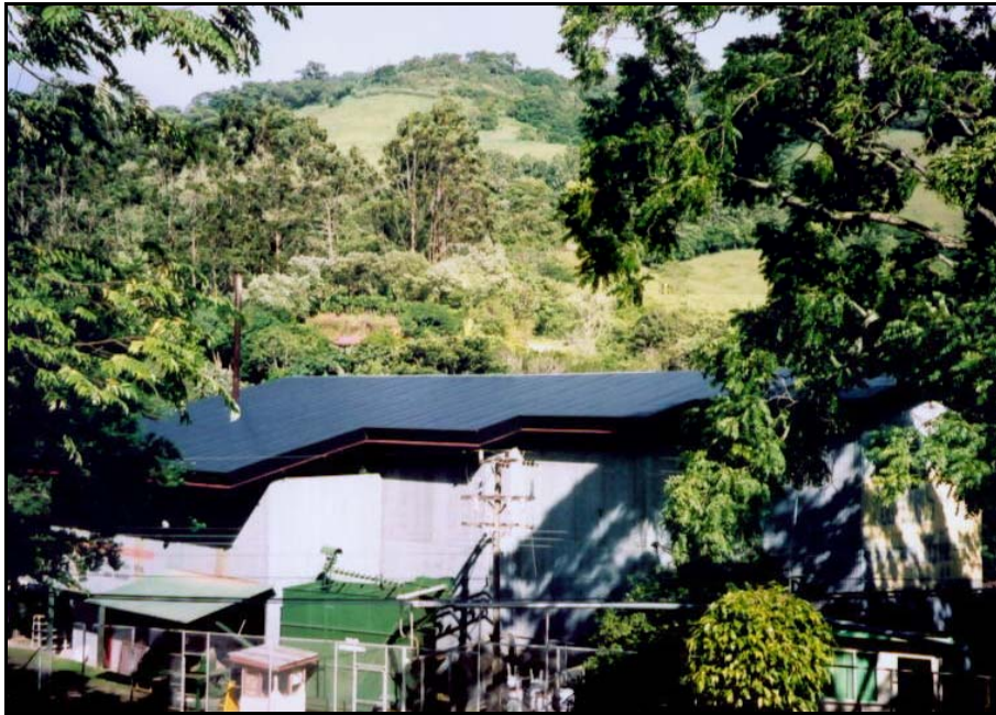
SOLARWALL® panels cover roof of coffee dryer in Tilaran, Costa Rica
